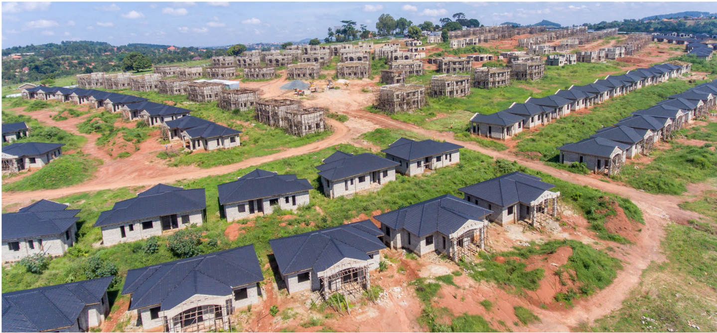
Construction ongoing at the Temangalo affordable housing project by the Fund
